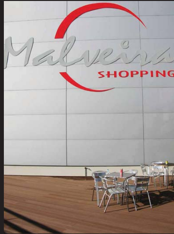
MALVEIRA SHOPPING | PORTUGAL terrace area
