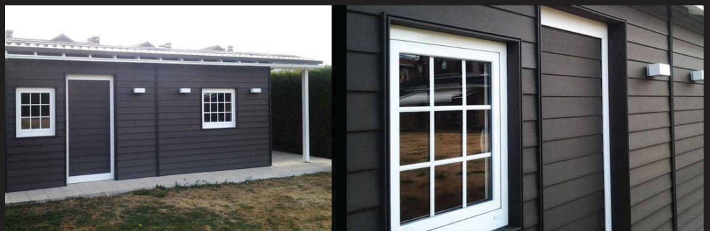
PRIVATE HOUSE | PAMPLONA | SPAIN house cladding
